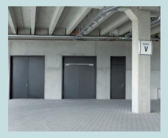
Doors which lead to the outside from storage areas (again with a matt black finish) were fitted with additional technical features: The doors can be easily actuated via a wall switch, resulting in the electrical revolving door leaf drive opening automatically.
