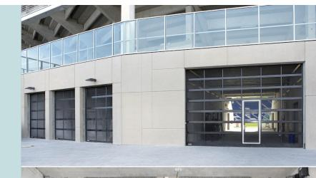
Outside broadcast vans in front of the stadium still receive live images even when the door is closed and locked. Visible on the right: The safety photocell which immediately stops the door when the light beam is broken.
