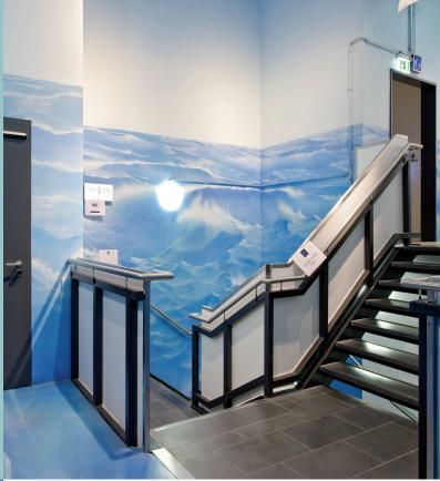
There are six staircases at the Klimahaus which can be used to evacuate the building in an emergency (in this case: Water from "The Elements" exhibition). Even the staircase has been incorporated into the design concept and elaborately decorated. The automatically driven door fades into the background. The sensor that monitors the swing range of the door is easily recognizable.
