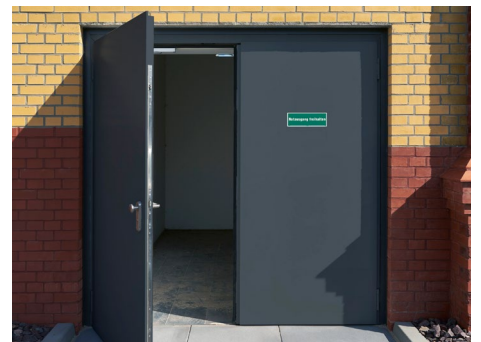
The emergency exits in the office tracts are also special: The safety doors (three-point multiple locking system, self-locking) are also equipped with full panic function. From the outside the doors thus protect the user from burglary, at the same time they are escape doors and can thus be opened to their full leaf width from inside and outside at any time.
