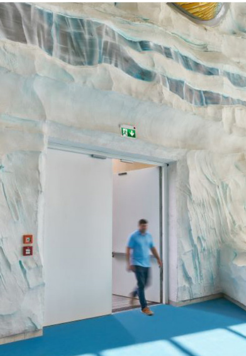
Large, double-leaf doors with panic function are used for the emergency exit.
