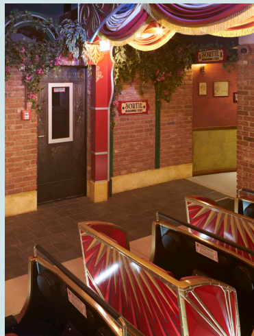
Glass inlets in the fire doors in the Moulin Rouge themed area provide necessary insight.
