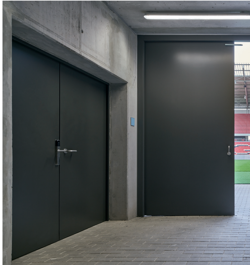
Hinged doors with the dimensions of an industrial door also leave room for large equipment and serve as an escape route at the same time.
