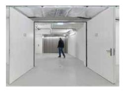
The majority of the 200 fire doors are used in the areas of the museum that are not accessible to the public. Here in the T90-2-FSA "Teckentrup 62" version, thick rebate, tested in accordance with EN 1634-1 (DIN 4102). The doors are connected to the smoke detection control panel and fitted with a release button. Other versions include panic lock, inactive leaf lock and holding magnets.
