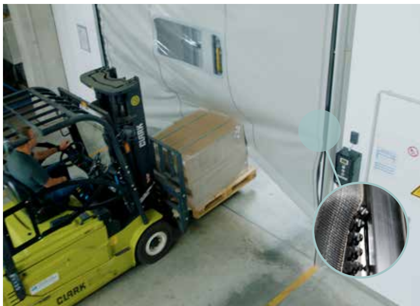
Protection of people and material through the integrated crash protection system with self-repair
