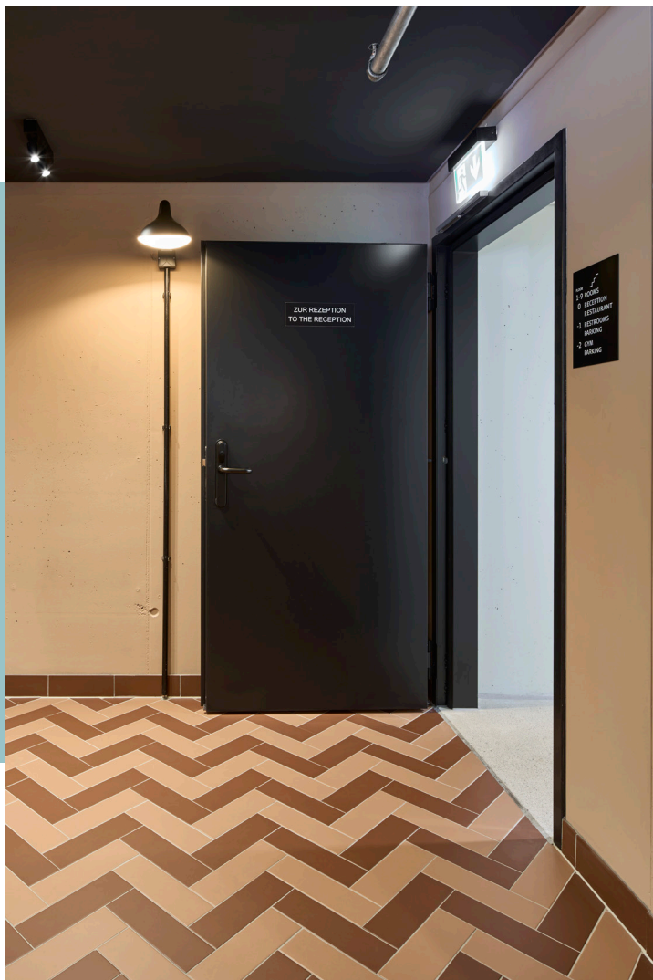
Doors with multiple functions can be found in the access routes, among other places: fire protection, escape route and aesthetics combined in one element.
