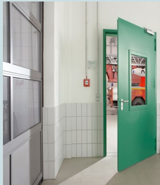
Clear view: The door to the vehicle hall is glazed to allow staff to see into the area into which the door opens.
