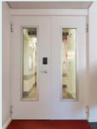
Glass inserts within the fire protection doors provide a clear view in the corridors.
