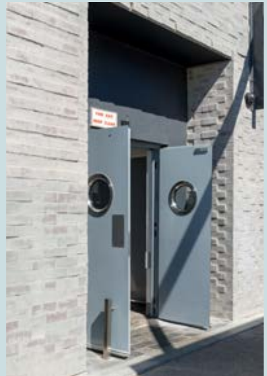
Even external doors, like the staff entrance, are partly equipped with bull's-eye.
