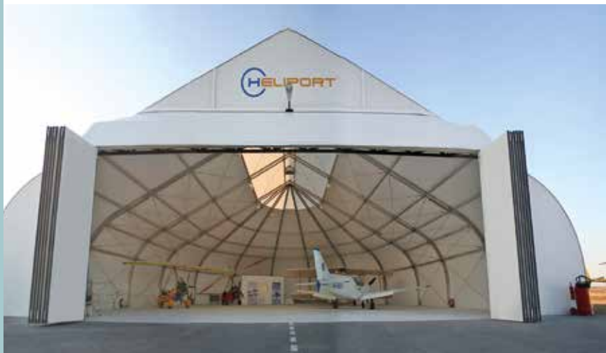
Twelve elements can easily be slid to the edge to open the hangar up wide.
